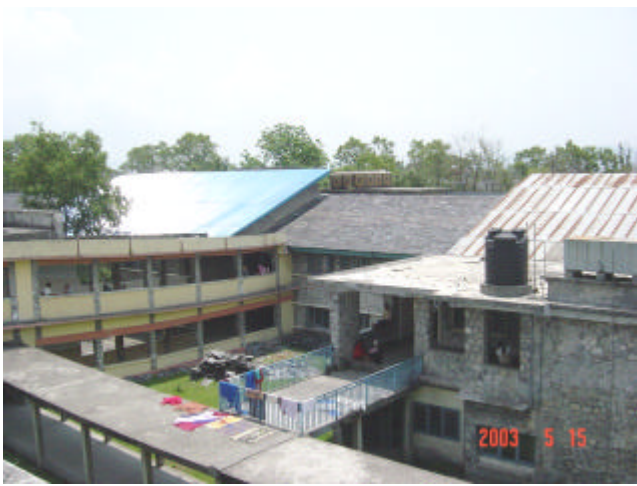
Photo 1: Buildings of different height, shape and structural properties connected with each other can cause severe pounding during earthquakes.
