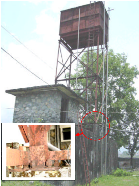
Photo 5: The base of an overhead tank; the bolts are not properly fixed and are rusted, the base is weathered.
