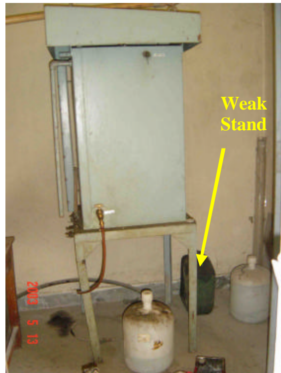
Photo 6: 300 litres fuel tank of the generator; on a weak stand without anchorage and lateral support.
