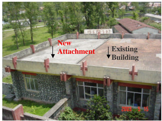
Photo 2: A new attachment to existing buildings with no seismic gap has made both the existing and the new building vulnerable.
