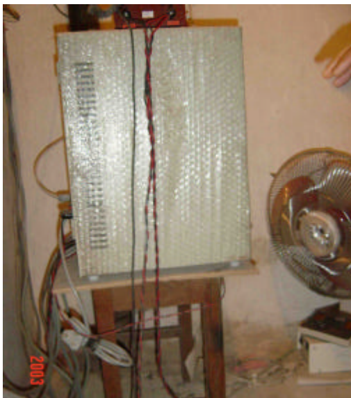
Photo 7: Communication equipment on a temporary type stand. It needs a proper stand with anchorage and fixing.
