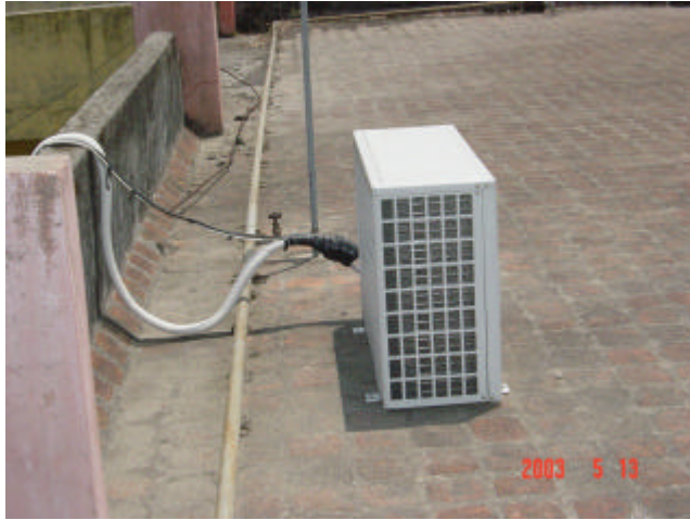
Photo 13: The air conditioning equipment for the OT is kept on the roof with no fixing.
