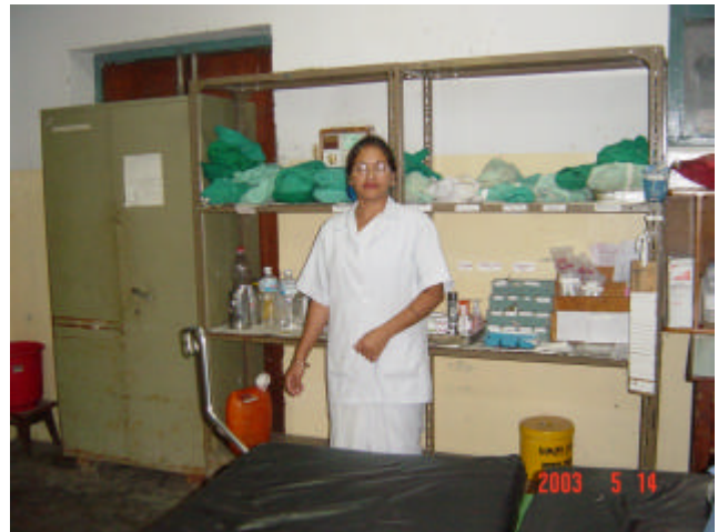
Photo 10: Cupboards and racks storing important equipment, medicines and chemicals are vulnerable because they are not fixed to the wall and strapped.
