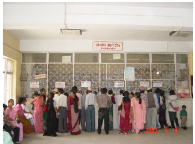
Photo 16: Window glasses or glass partitions are life safety hazards and need plastic lamination.
