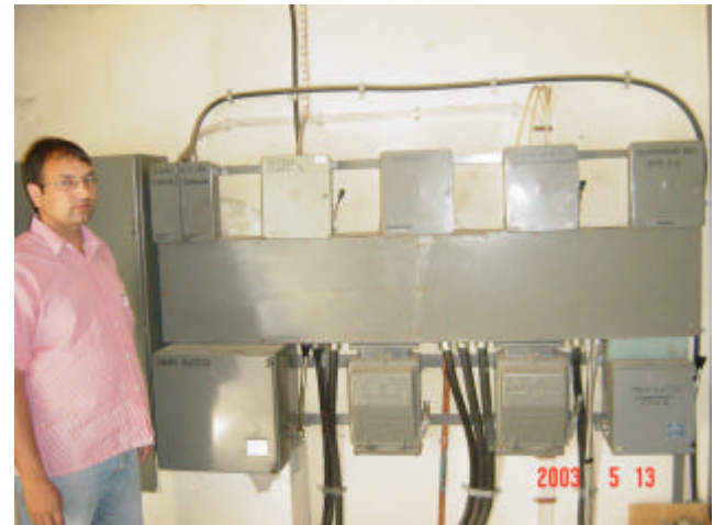
Photo 8: The main board for electricity distribution within the hospital; properly anchored on the wall and with low vulnerability.
