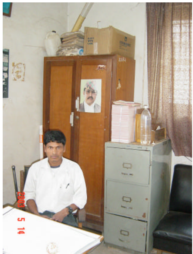
Photo 12: The cupboards and racks near working stations in the administration and other places of the hospital can be life safety hazards.
