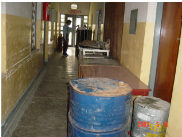
Photo 15: Cupboards and other objects in the corridors can block the exit ways during earthquakes.
