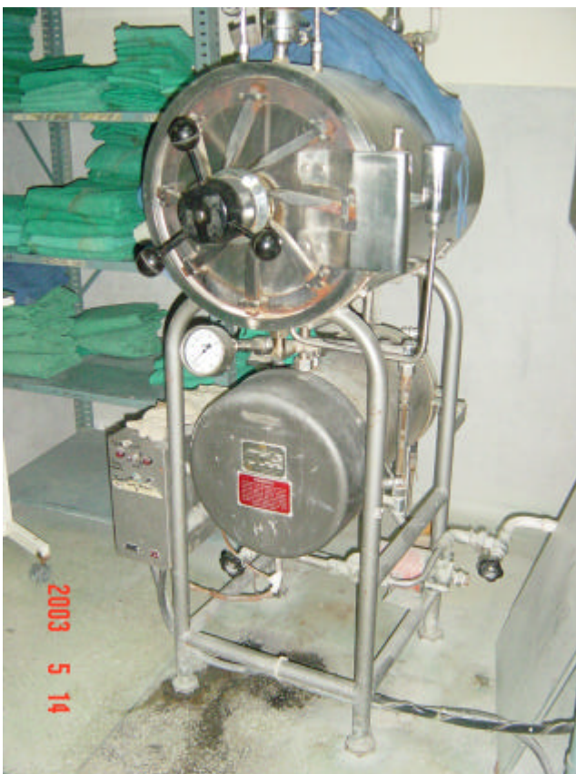
Photo 11: Autoclave machine needs anchorage at the base.
