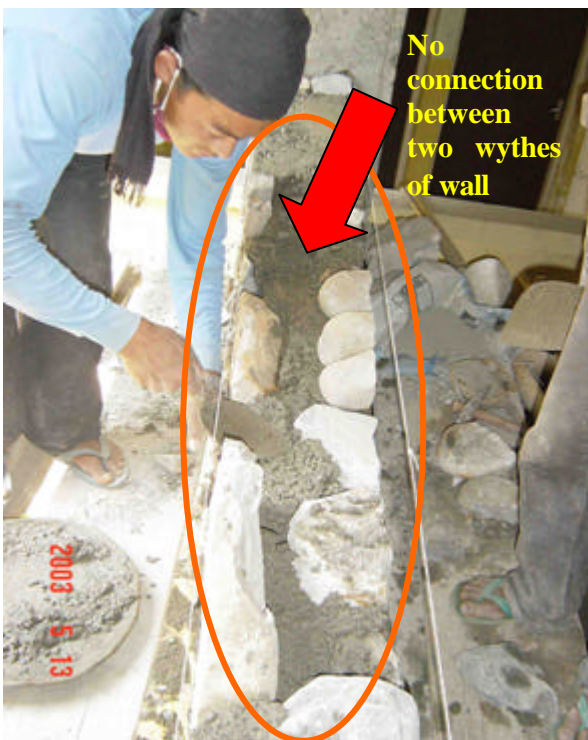
Photo 3: A stone masonry infill wall construction in the new building. There is no proper connection between the stone units making it a very vulnerable wall. The mortar used is 1:6 cement: sand mortar.
